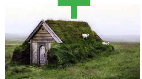
Above: "A small turf house in Fellabær, Iceland: Icelandic turf houses are the product of a difficult climate, offering superior insulation compared to buildings solely made of wood or stone, and the relative difficulty in obtaining other construction materials in sufficient quantities. Turf, or earth acts as thermal mass, making it easier to maintain a steady indoor air temperature and therefore reduces energy costs for heating or cooling."
